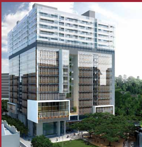
Brisbane Supreme and District Court Building.
